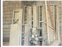
#3: Power Climber Suspended Platform
