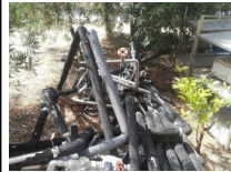
#16: Lot of Fixed Pipes
