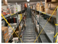
#20: Electrical Equipment Warehouse
