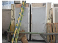
#49: Chemical Toilet and Tanks
