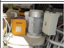
#52: N. 2 tanks with mixer
