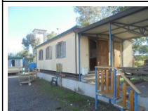
#58: Prefabricated structure used as a canteen
