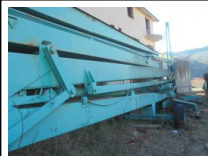
#1: Self-Elevating Crane and Construction Equipment
