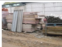
#1: Equipment for Construction Site
