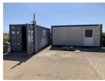
#21: Container and Office Box
