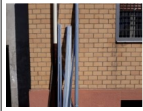
#14: Construction Equipment -B
